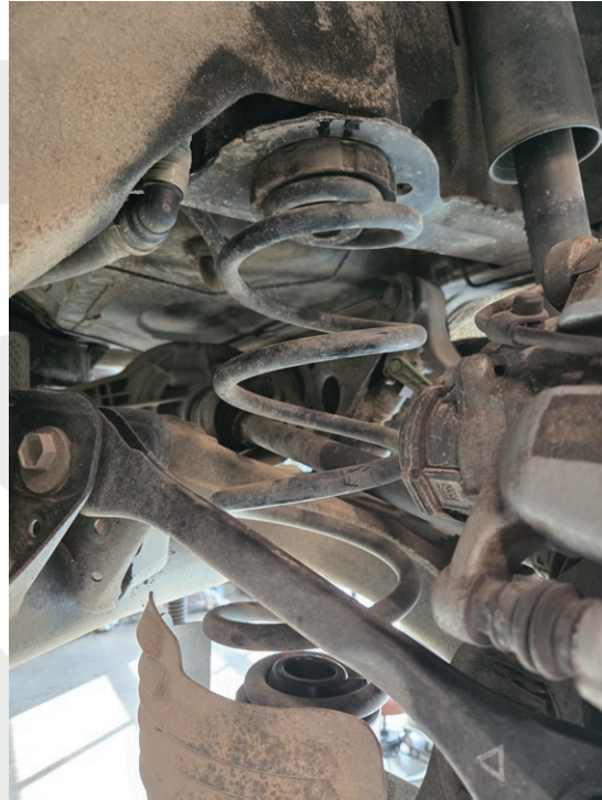
Reinstall coil spring in vehicle - be mindful of orientation of spring on spacer. Use pole jack to lift subframe back into place.
